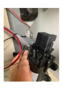
21. I like to mount the pump above the sink cabinet shelf as close to the back so that the hose doesn't kink. The pump can be mounted just about anywhere under the sink cabinet. Here are a few examples
