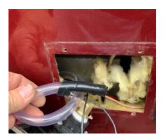
31. Insert tank water line with filter into bottom of new fitting. you may have to unbend plastic hose to be a bit more straight. Hose should curve into the bottom corner of tank.
