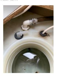
32. Connect new water line to the new water tank connecter.
