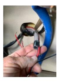
20. Attach pump ground to pillar with the cabinet screw and connect hot power wire to either the yellow hot faucet wire or another hot source.
